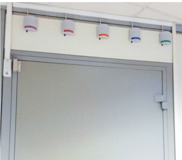
Five optical signals installed above the door
