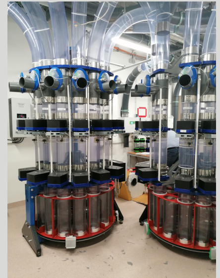
The picture shows two revolver. These are usually stored in the technical room of the building.
