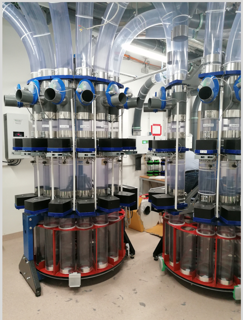
The photo shows our revolver. This is usually housed in a technical room in the basement of the building.
